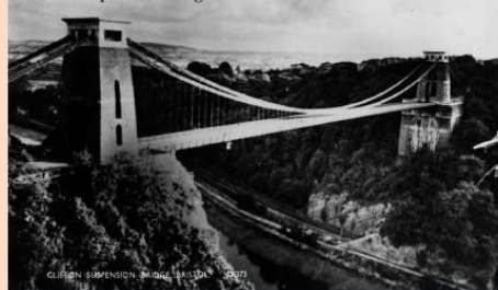
Clifton Suspension Bridge
