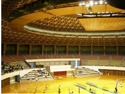
Photo 2: Conical steel framed shell (Zero Gaussian curvature)
