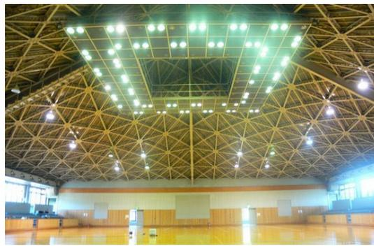
Photo 3: Hyperbolic paraboloidal steel framed shell (Negative Gaussian curvature)
