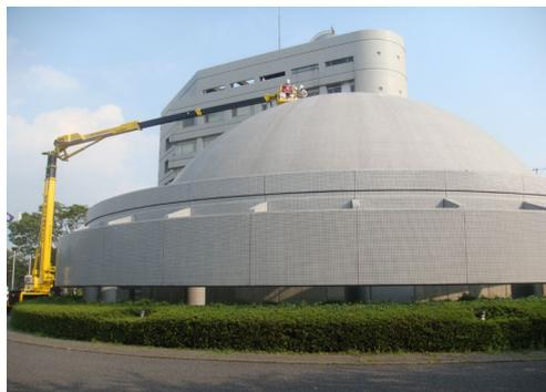
Photo 1: Spherical concrete shell (Positive Gaussian curvature)
